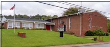
<< Street front view of St. Paul Lutheran Church 412 5th Street, New Haven, WV. Fellowship Hall is behind church.
